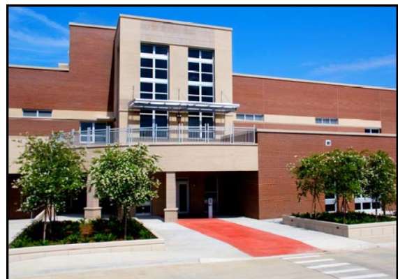
Public Safety Complex
